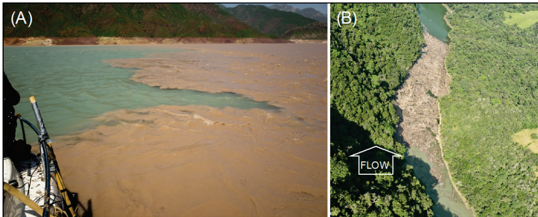
Figure 8. (A) Turbid water plunging into Nurek reservoir, Tajikistan. (B) Accumulation of floating debris at the density current plunge point in Miel-1 reservoir, Colombia (photos G. Morris).
