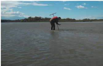
b. Lewis and Clark Lake, SD – Large sediment loads from tributaries have resulted in at least a 30% loss in total storage capacity (USACE, 2013). The upper reservoir is now so shallow that boats can be beached in the middle of the lake (upper left photograph) and the reservoir can be waded (lower left photograph). At least part of the City of Niobrara, NE had to be relocated because of the upstream growth of the sediment delta even though it was upstream from the reservoir pool (right photograph).
