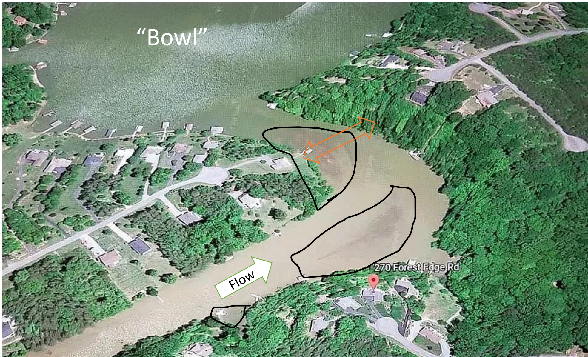
2017 Upper Gills Creek Identified Area with Sediment accumulating, severely obscuring the opening downstream
