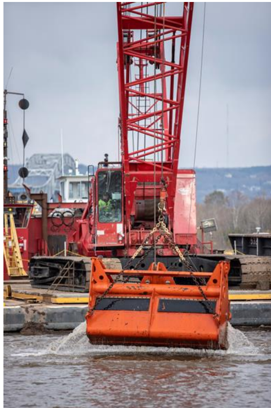
Figure 6 Mechanical Dredge Consisting of a Crane Using a Clamshell Bucket
