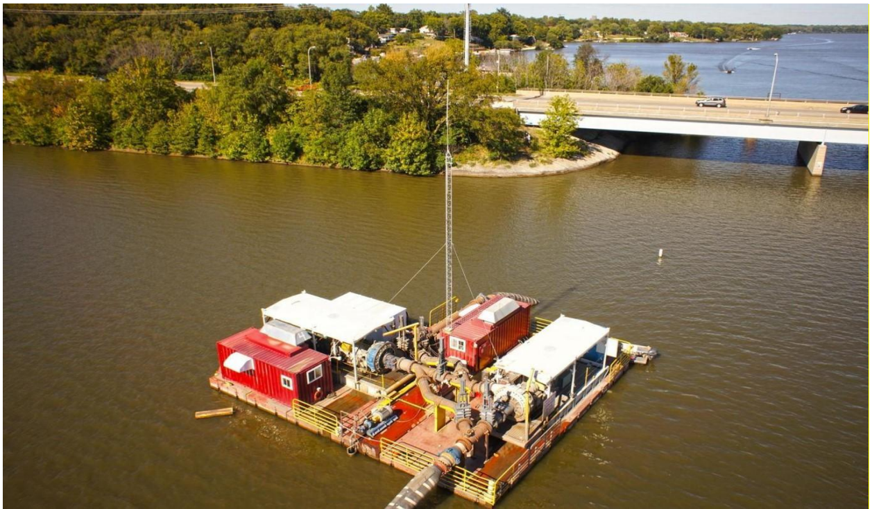
Figure 12 Booster Pump Station at Lake Decatur, Illinois
