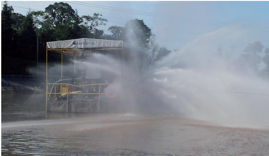
Figure 24 Modified Hydrosuction Water Jetting Array
