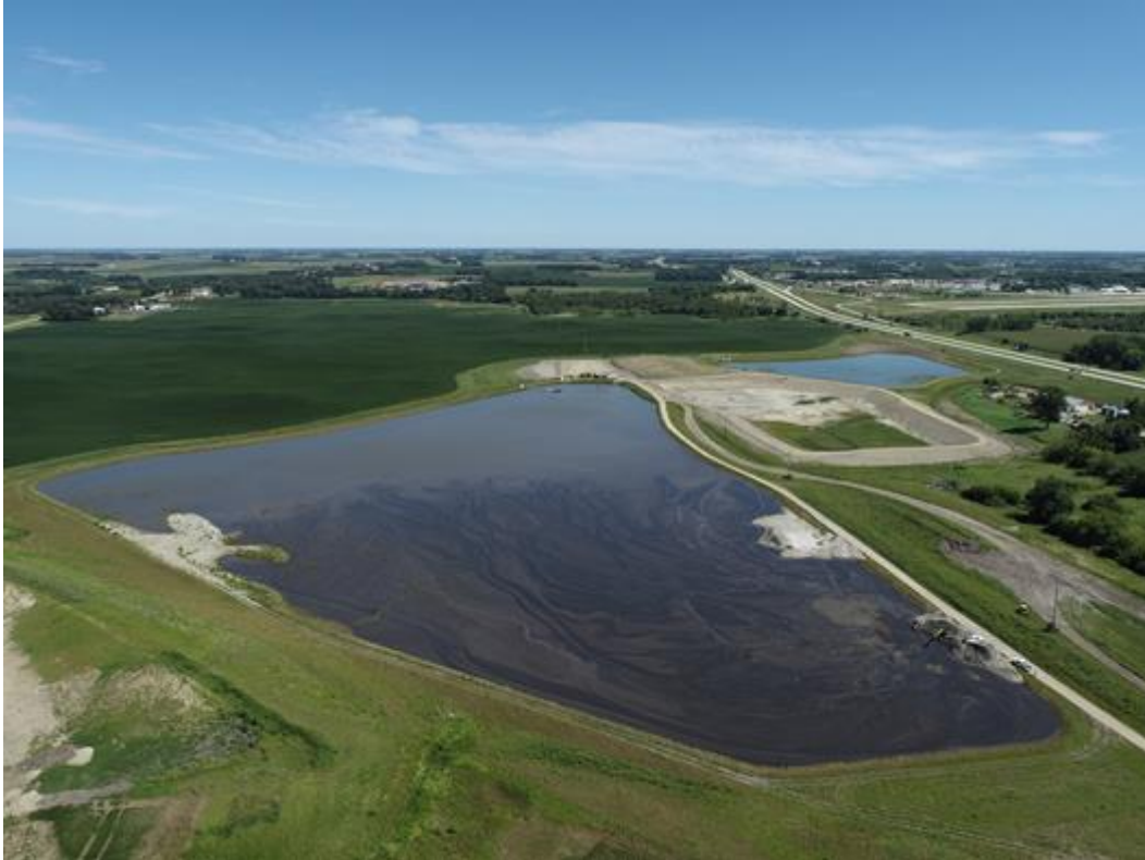
Figure 16 Example of Confined Upland Placement Area for Sediments
