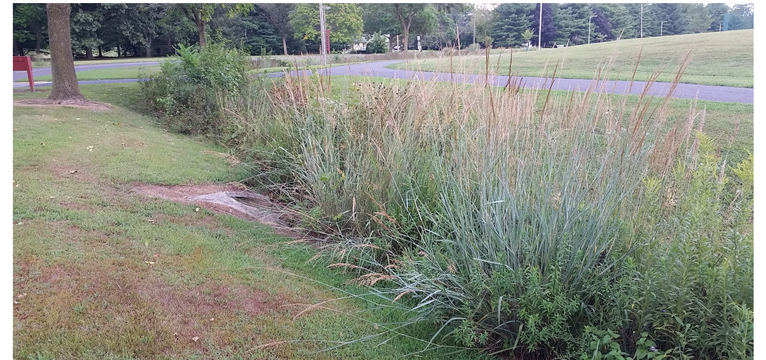
Example of a vegetated channel; Sewell, New Jersey; Designed by Princeton Hydro
