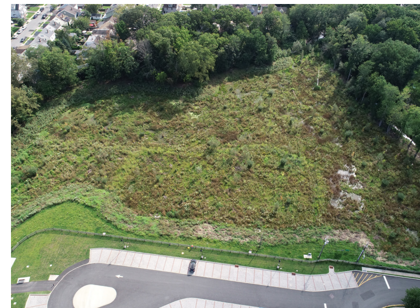
Constructed wetland; Bloomfield, NJ; Designed by Princeton Hydro
